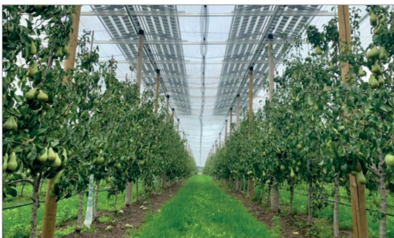
Figure 1. Pilot agri-PV in an orchard at Bierbeek, Belgium, illustrating the benefit of bifacial cells for high-transparency modules placed at a high elevation.
