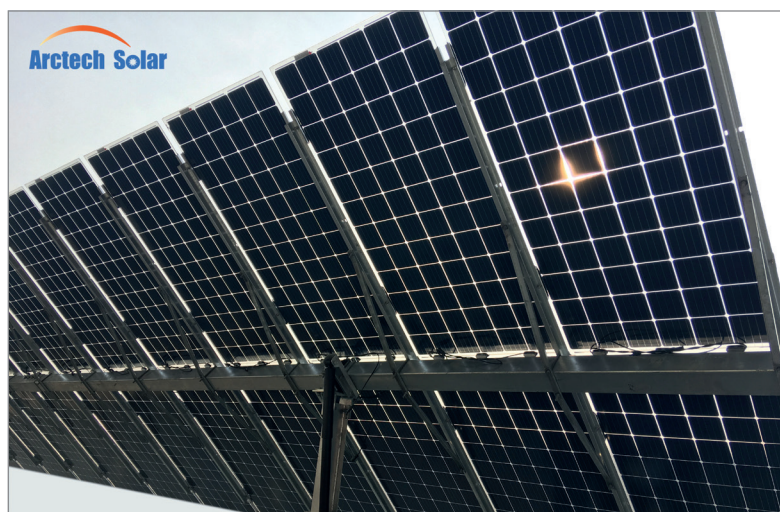
Figure 3. Independent horizontal single-axis tracker from Arctech Solar, designed for bifacial modules [145]. The modules are fixed using aluminium elements at the module edges, overlapping with the long purlins to avoid covering the back of the bifacial modules. Junction boxes at the module edges in such a system, as shown, can be integrated without shading caused by cables. (Source: Arctech Solar.)
